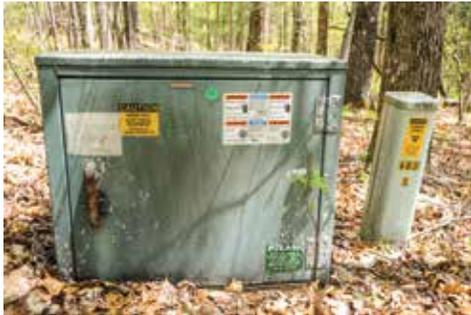
*Figure 6 – Electric transformer and telephone junction box provides service to lots 9 and 10*
