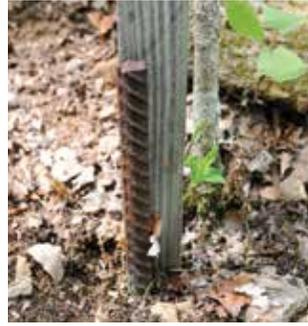
Figure 2 – left, Steel rod marks line between lots 39 and 40.
